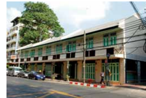
Figure 11. Khao Hong shophouses before rehabilitation (source: CPB)
