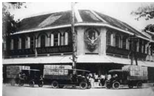
Figure 5. Shophouses of Talat Ming Mueang before redevelopment (source: National Archives)
