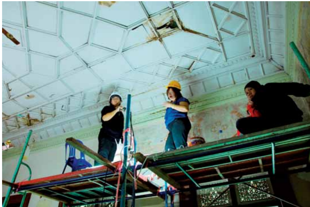
Figure 13. CPB staff at site investigation (source: CPB)
