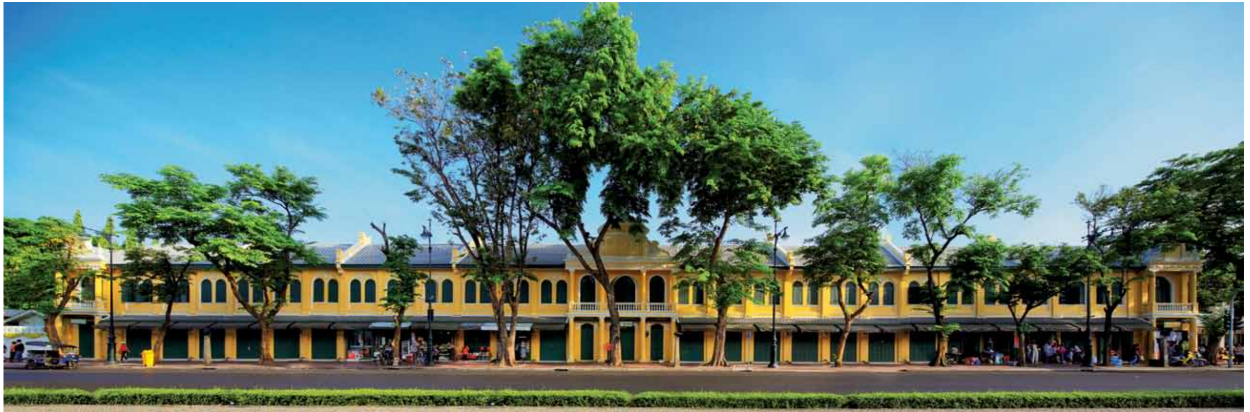
Figure 19. Na Phralan as an example of shophouse restoration under matching funding program (source: CPB and Association of Siamese Architects)
