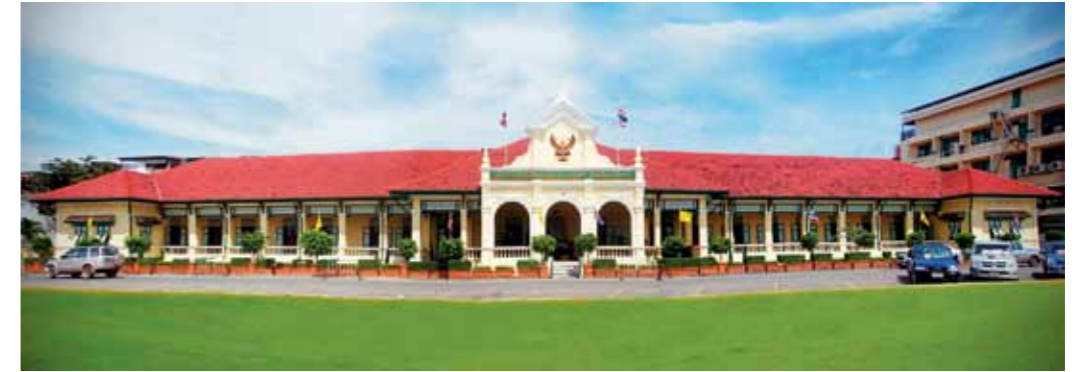
Figure 17. CPB Regional Office in Chachoengsao (formerly Prachin Provincial Hall) (source: CPB)
