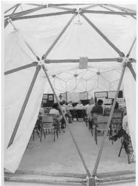
Figure 5. Demountable geodesic dome prototype, devised by R. Buckminster Fuller and Shoji Sadao in 1981, for covering Ban Chiang and other sites.
